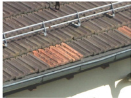
Figure 10: Roof with recently substituted bricks [13]
